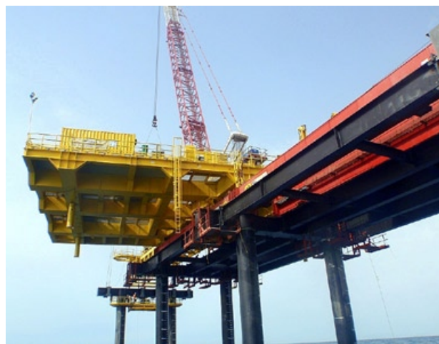
Moving construction crane platform
